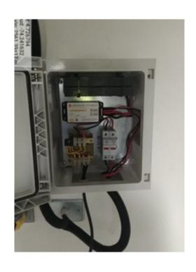
Synergistic remote monitoring units for on/off potential inspection campaigns that allow a better understanding of the behavior of the PC system.
